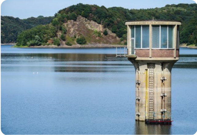
Drinking water reservoirs
